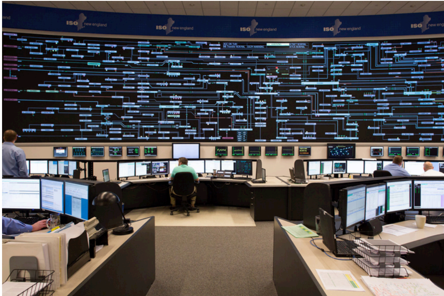
ISO New England Control Room
